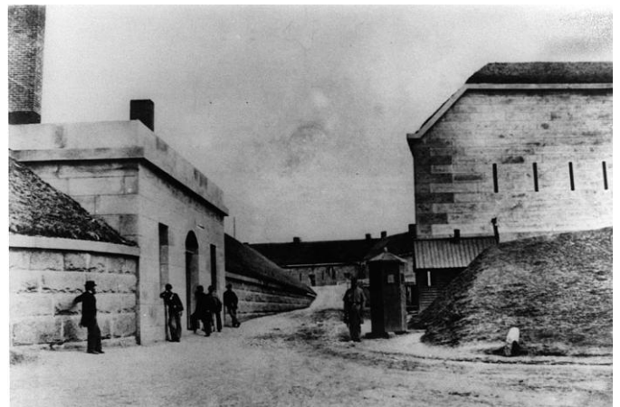
The guardhouse (left) and sentry box (on right) at the entrance to Fort Warren about 1861. The fort is located on Georges Island at the entrance to Boston Harbor.
